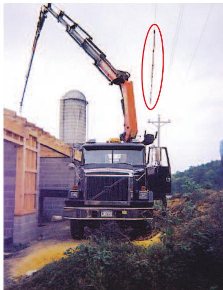
**RUBBER LINE GUARDS:** Special cover up material used to cover energized lines to prevent an accident, is placed on the wires by the co-op.
