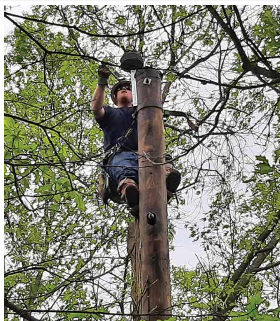
REPLACING POLES: Crews are working in the Waterfall Hill area replacing poles. Lineman Kyler Fink is working on tying in the phase wire.
