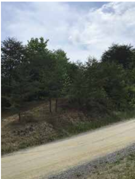
THROUGH THE TREES: An old power line runs through a group of pine trees to feed one of the homes in the development.
