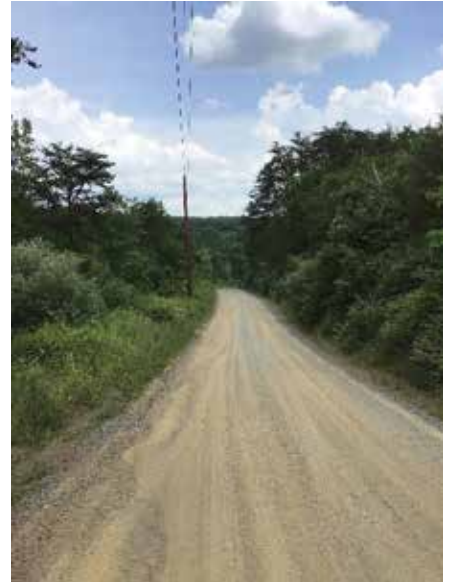
PROJECT COMPLETED: This section on Waterfall Hill is completed and ready for years of reliable service.
