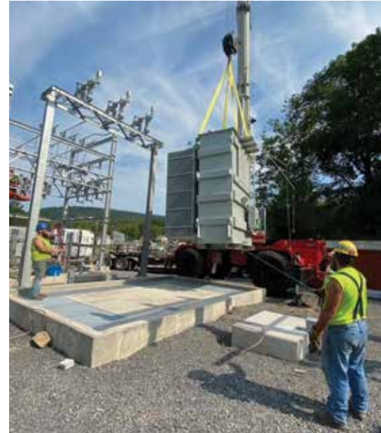
A WATCHFUL EYE: Crews set the Bay 1 transformer in place at the new substation site.
