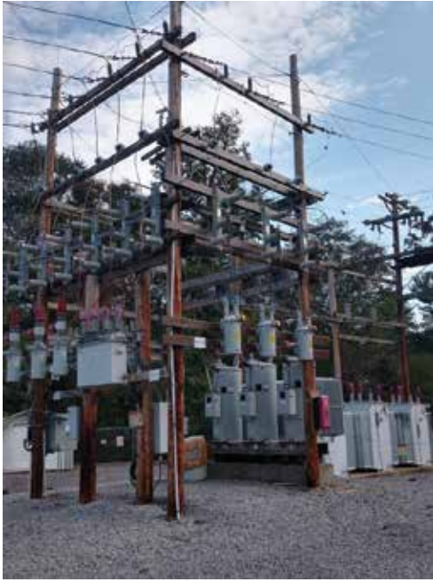
OUT WITH THE OLD: The wooden Waterfall substation, above, served cooperative members in Huntingdon and Fulton counties since 1975. It was recently replaced with a new steel substation at the site.
