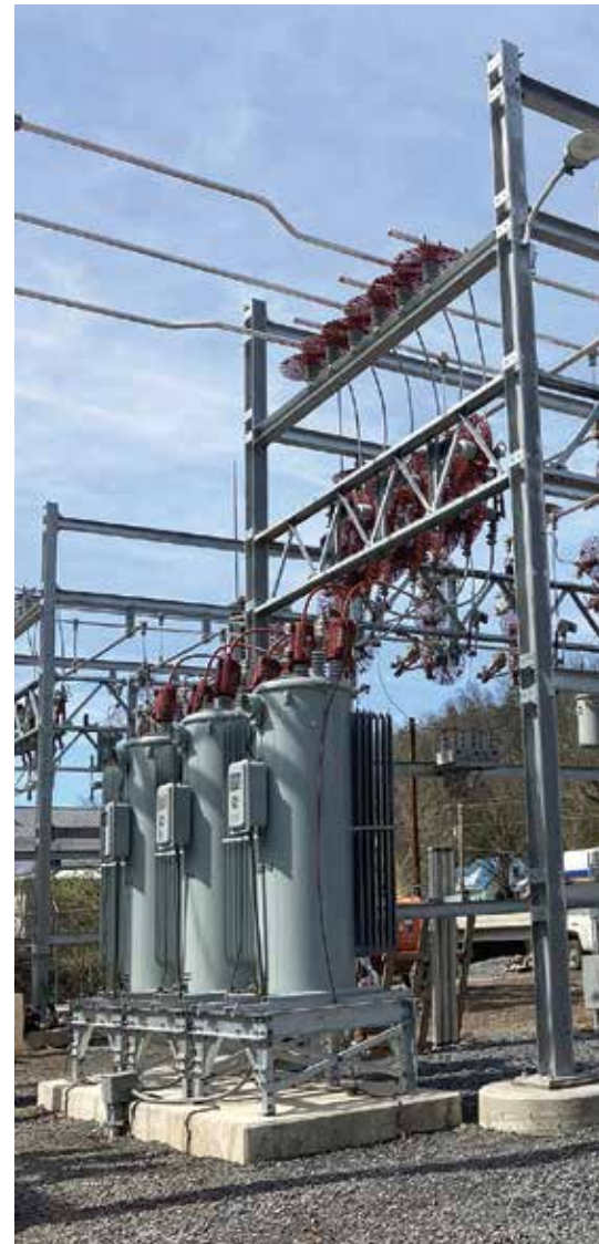
A WATCHFUL EYE: Crews set the Bay 1 transformer in place at the new substation site.
